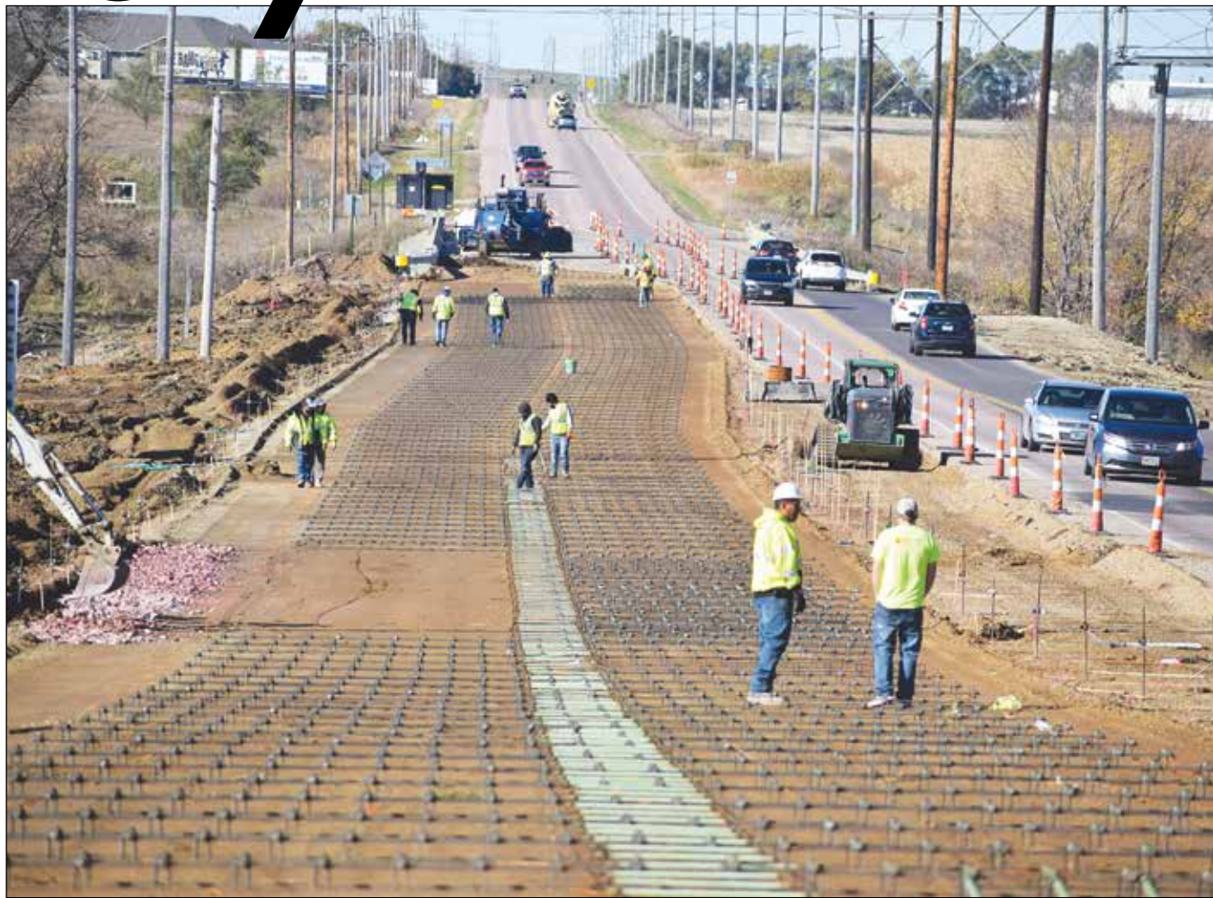
Work progresses last fall on the Holly Boulevard Crossing just west of the Sioux Boulevard intersection.
