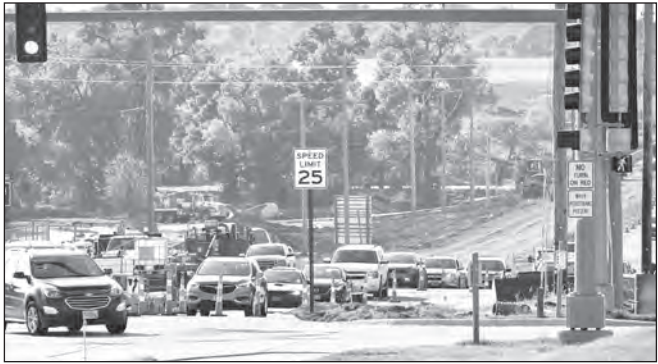
Jamie Hult/File photo The north side of Holly Blvd. opened after five weeks of construction, but sewer and storm sewer work continues on the south lanes, as does the 25 mph speed limit through the construction zone.
